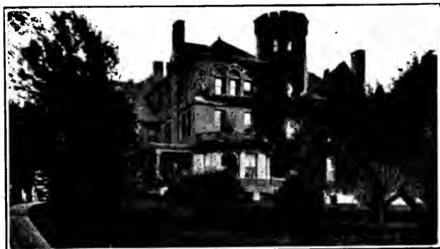
RESIDENCE OF THE LATE S. D. COYKENDALL.
